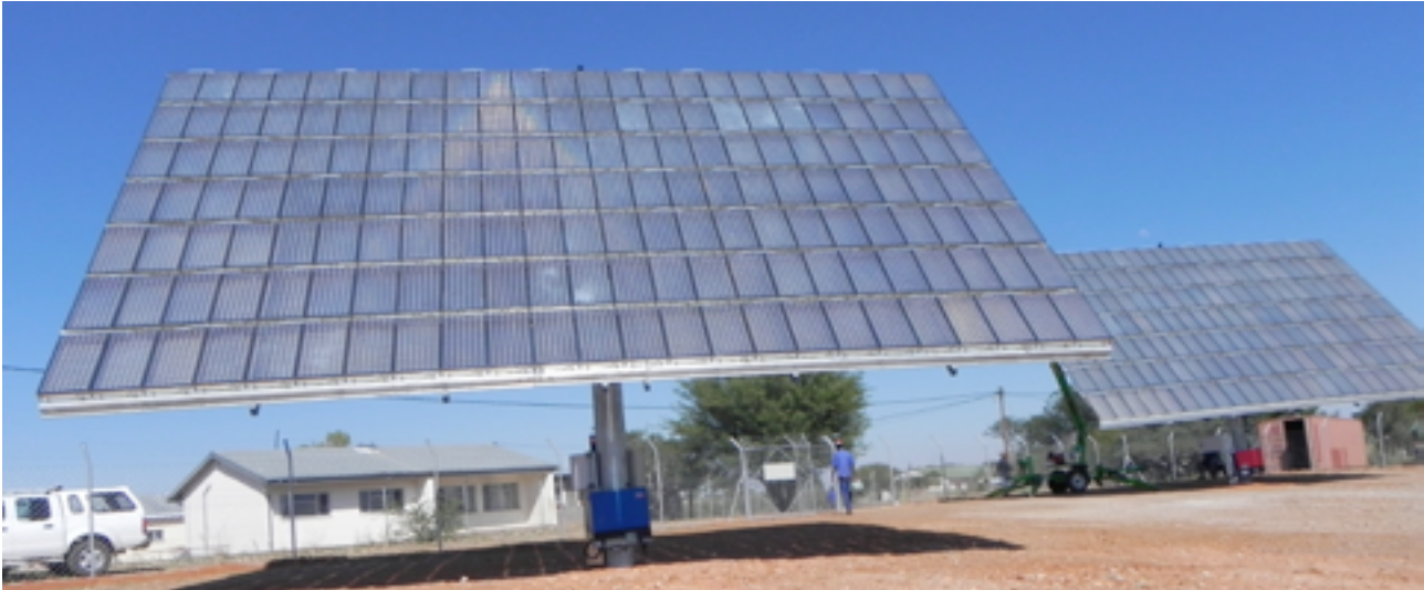
The Usib (26 kWp) Concentrator Photovoltaic Plant.
